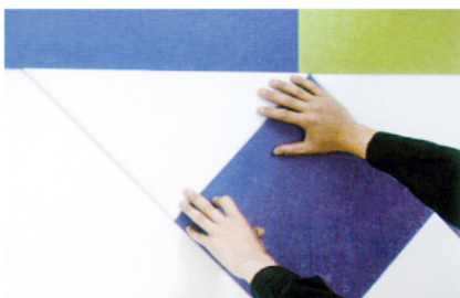
◆ 將打好膠的吸音板按墨線上牆 Installation.
