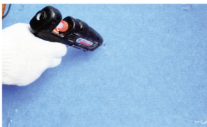
◆ 給吸音板打膠 Apply adhesive.
